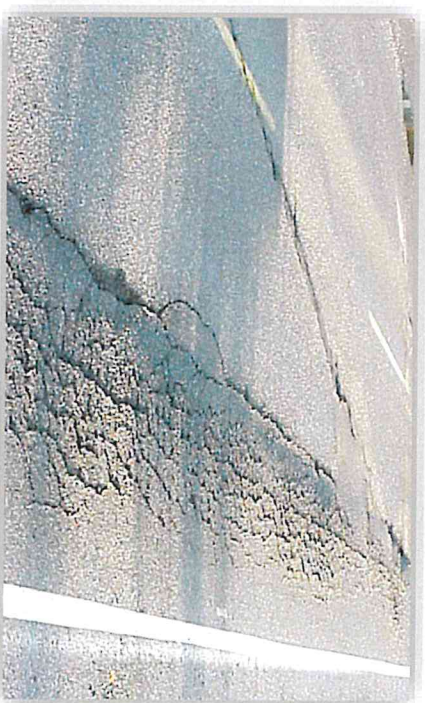
Base Failure
