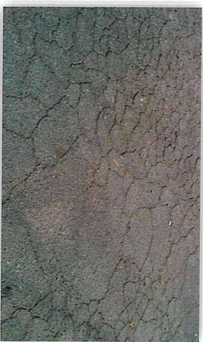
Alligator Cracking
